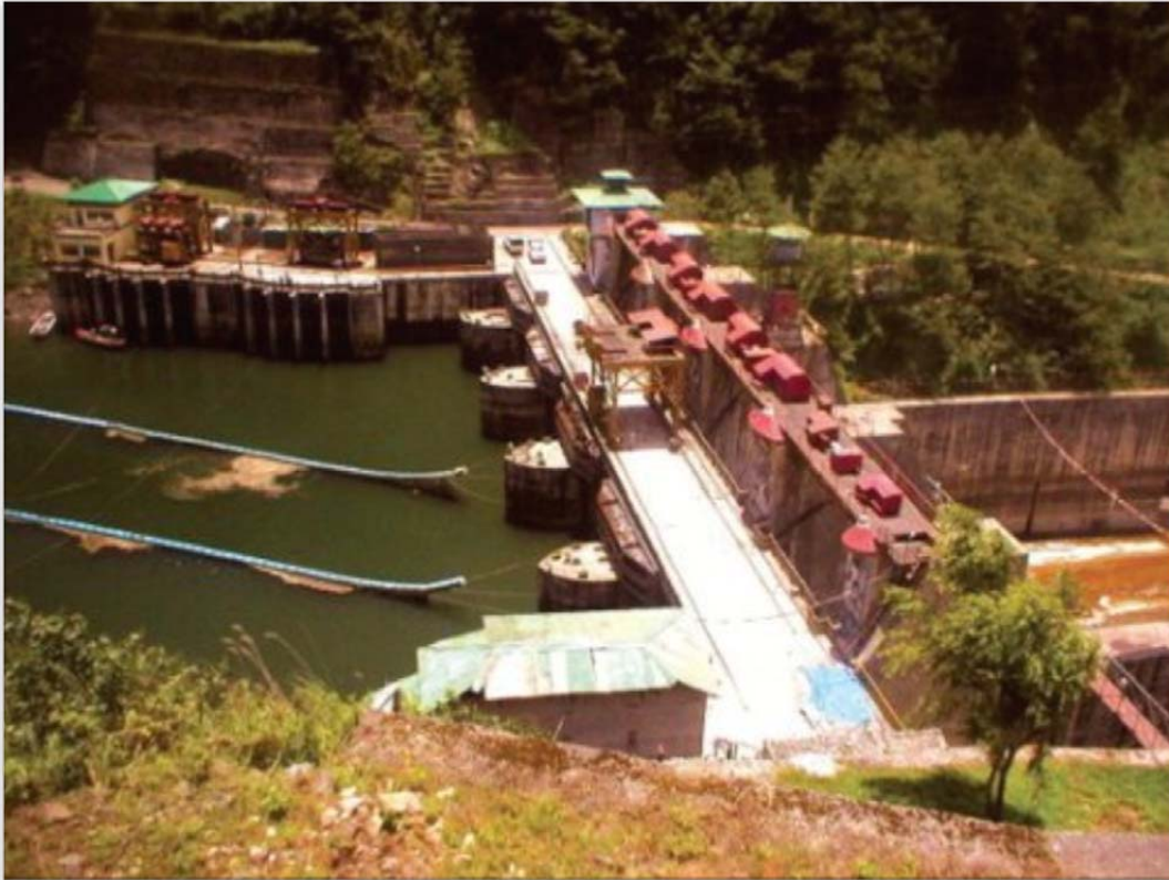
1986 – Chukha Hydropower Project, Bhutan
